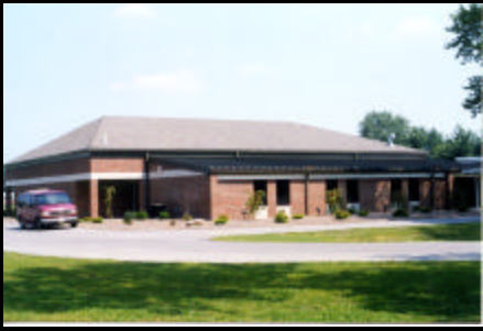
Above: Echo Meadows newly finished rectangle structure.
