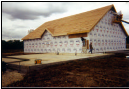
Above: First Presbyterian Church of St. Mary's, OH after assembly
