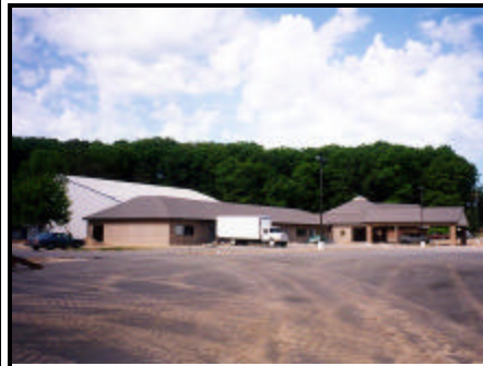
Above: Lakeshore Baptist Church during construction.
