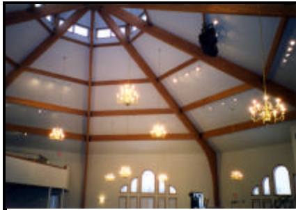
Top: Revival Fellowship shown with it's cupola and 18' sidewall. The exterior is finished with green shingles and beige dryvit.
