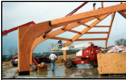
Above: Assembly of New Testament's new 96' octagon
