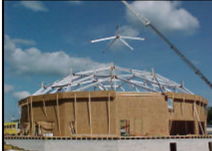
Top: Open Bible Tabernacle's 100' square in Marietta, Georgia Bottom: Setting beams for Brookhaven Wesleyan Church's 110' dome in Marion, Indiana
